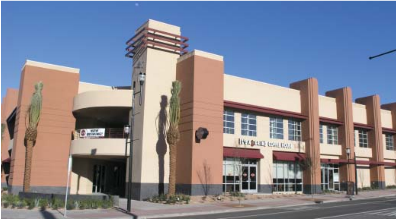
Water Street South, one of Henderson's top redevelopment projects, is revitalizing the downtown area.
